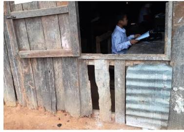
Poor structural design and the passing of time had caused the buildings to become quite deteriorated, with holes in the walls and roof and cracks in the foundation
